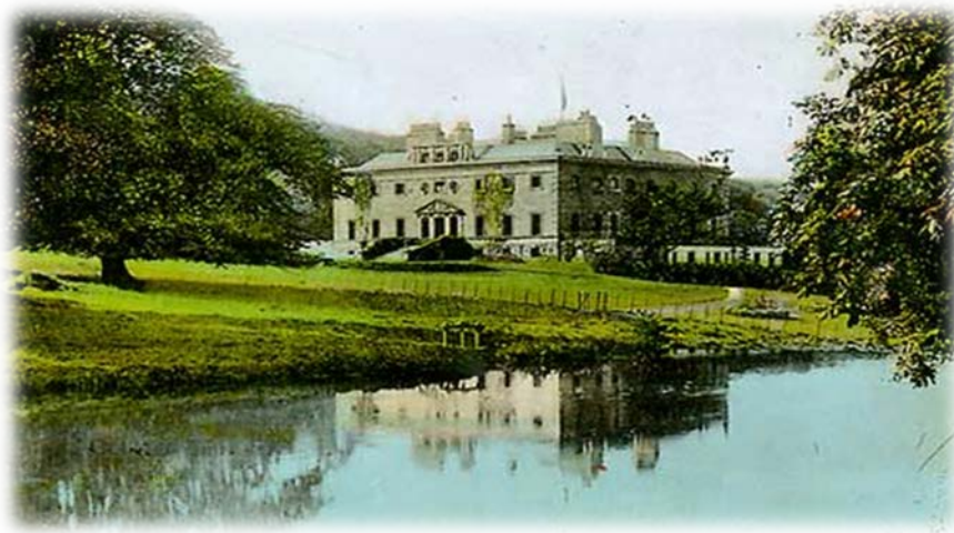
Figure 11 Westport House (The Database of Houses , 1999)
